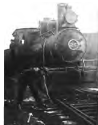
Fig. 4. Dangerous Switch Arrangement.
